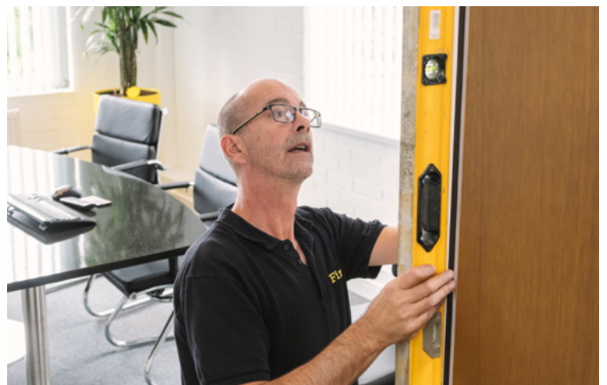
Fire doors will only protect your building if they're compliant.
