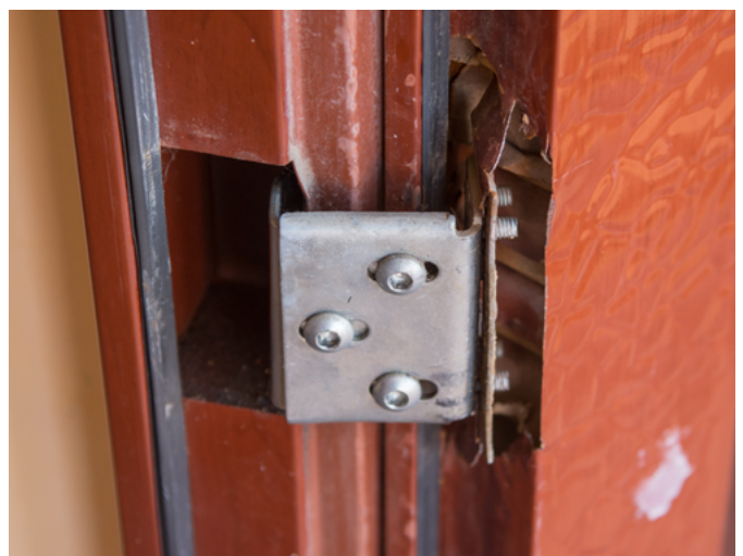
Fire doors will only protect your building if they're compliant.
