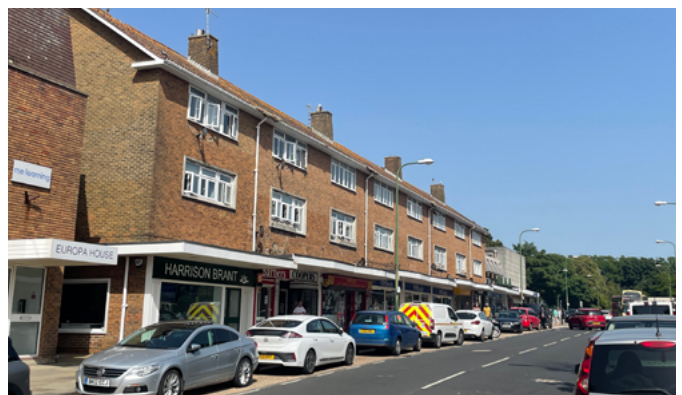
Southwick, East Sussex, where a change in legislation required installation of compliant fire doors
