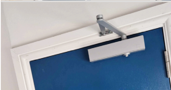
(Top left) The correct plugs and labels were added to the door to show certification. (Top right) Intumescent seals prevent smoke and fire spreading in the event of a fire. (Bottom) An appropriate door closer was installed.
