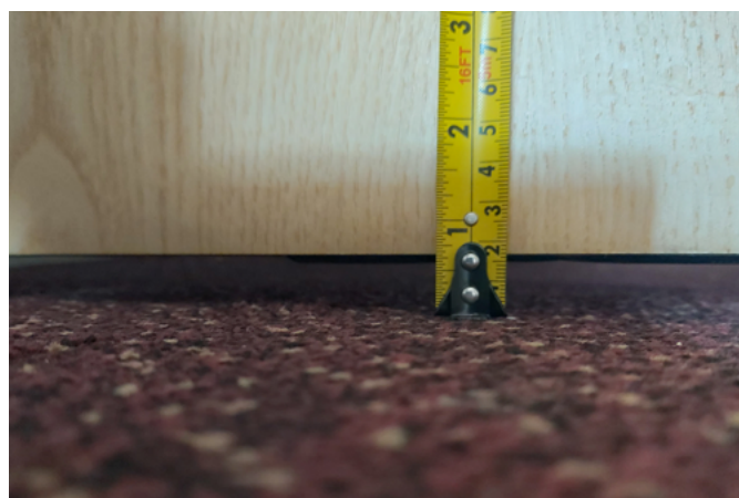
Compliant fire doors should have gaps around the frame of no less than 2mm and no more than 4mm.
