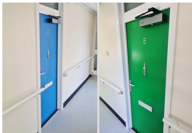
Freedor: removing the effort involved in opening and closing heavy fire doors.
