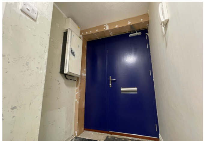
The complete doorset install from the inside of the property.
