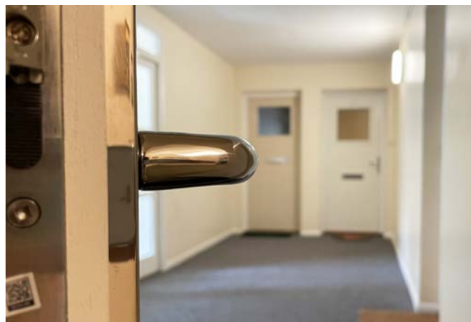
All news doors were fitted with fire-rated ironmongery
