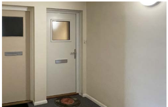
One of the new doors installed at The Priory
