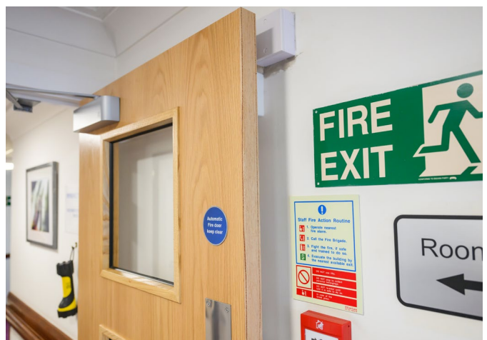
One of 126 new doors installed at Oakland; an American oak veneer doorset with three vision panels & ironmongery.
